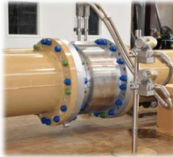
Figure 19: Typical Liquid Ultrasonic Meter Installation
