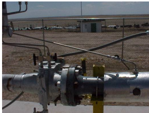
Fig 4. Orifice fitting with natural gas flow
