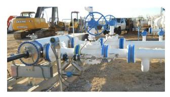
Figure 15 – Inferred Prover Installation
