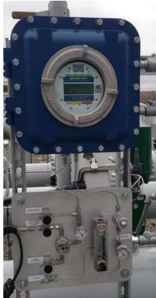
**FIGURE (3)- HCD5000™ On-line Hydrocarbon Dewpoint Analyzer**
